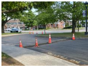
Parking lot repairs.
